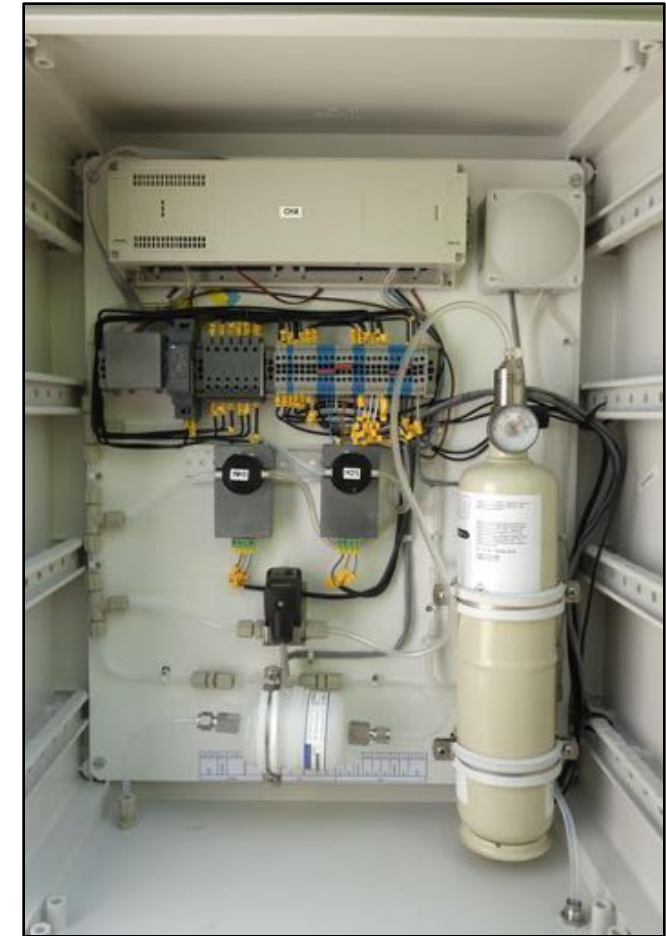
Dynamic gas sampling system with automatic zero gas calibration
